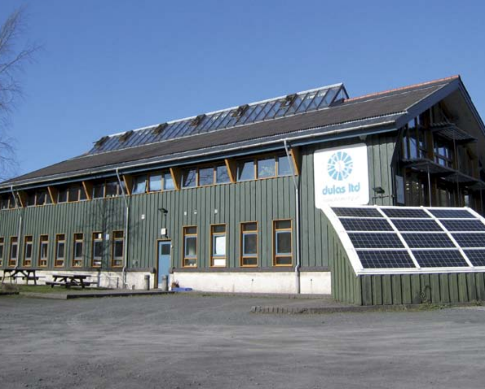
Dulas offices, Dyfi Eco Park, Machynlleth. Courtesy of Dulas Ltd
